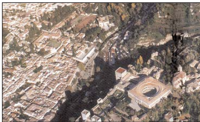
Courtyard network, Granada, Spain
